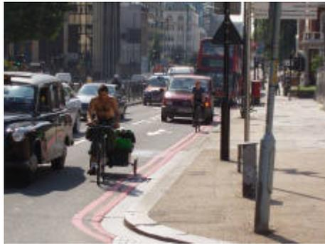
The push-buttons at the signalised pedestrian / cyclist crossing at Upper Ground are only partially used. Cyclists apparently prefer not to wait at the signal when cycling on the southbound cycle lane across the bridge, but merge into the traffic across two driving lanes. The layout with cycle lanes do not prevent the merging manoeuvres.
