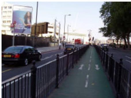
The carriageway of Blackfriars Road on this short section between Upper Ground and Stamford Street is narrow on the west side. This provides poor conditions for the cyclists, and the cyclists actually hamper cars moving forward in the outer drive lane. This is critical here (creates frustrated motorists) because cyclists are slow upwards towards the bridge.
