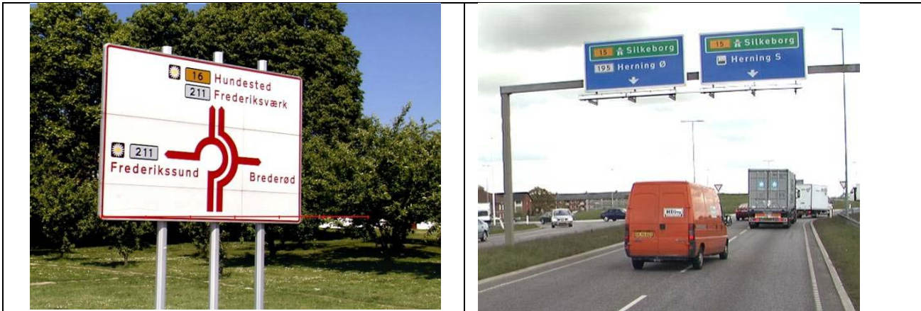
FIGURE 7. Two different signing concepts at the entrance to the 2-lane roundabout. Left – “lane use-sign” and right – use of portals.
