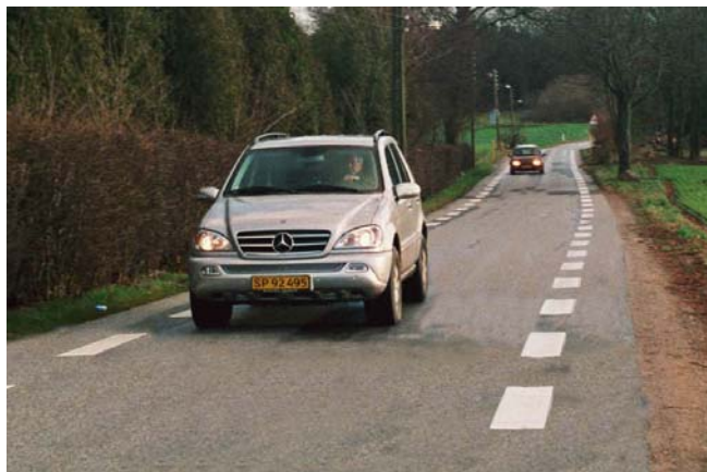
Figure 2: After situation. One central driving lane
