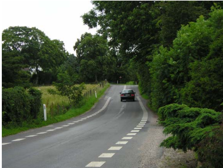
Figure3: Centre line marking is remained in curves when "stop sight distance" is too short.
