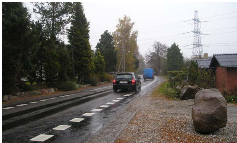
Figure 5: In meeting situations drivers give way to on-coming cars by crossing the intermittent edge line a little bit as intended.
