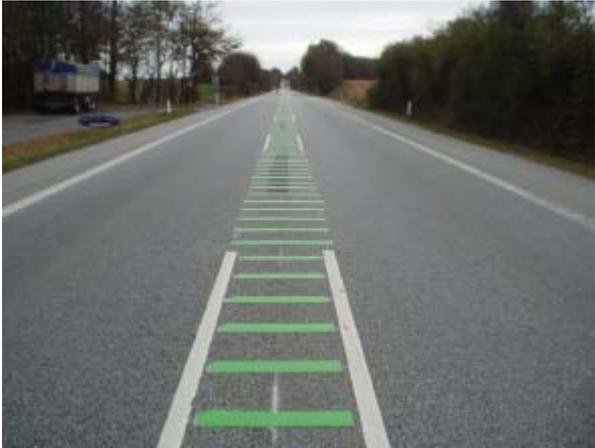
Figure 5.1a: Centre line marking – design A.
