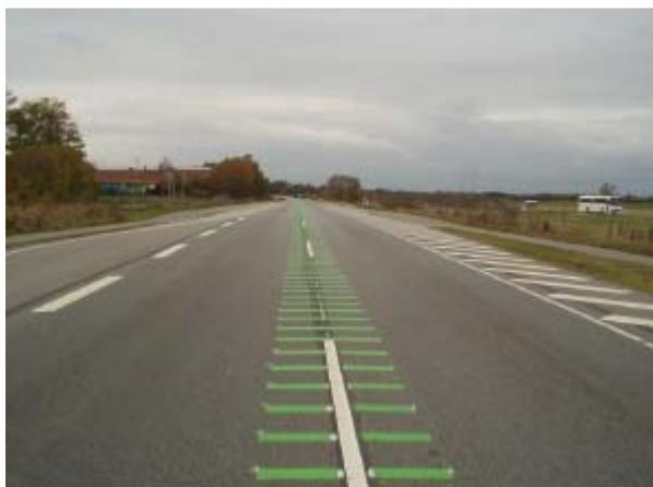
Figure 5.1b: Centre line marking – design B
