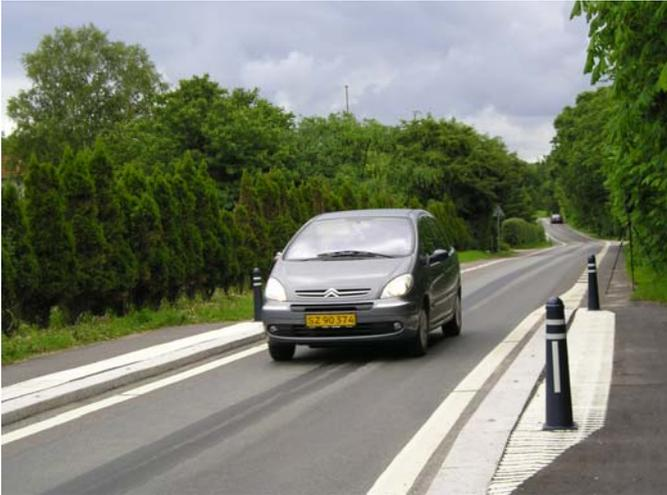
Figure 9: Speed reducer designed as narrowing with only one central vehicle lane
