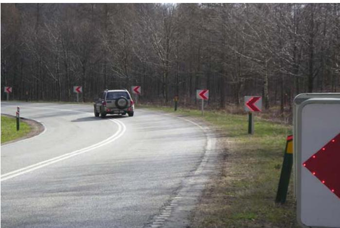
Figure 11: Chevrons in dangerous curves illuminate if speed is too high
