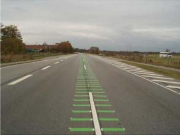
Figure 6: Centre line marking – design B
