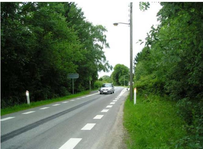
Figure 8: "2-1"- cross profile with one central driving lane
