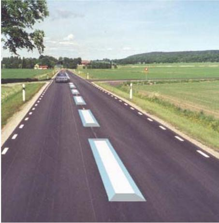
Figure 3: Three-dimensional markings
