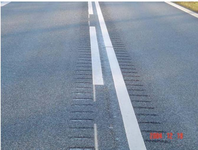
Figure 7: Rumbling marking along centre lines
