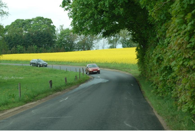
Figure 3: If the road is a minor road in a rural area, we expect it to be narrow and winding
