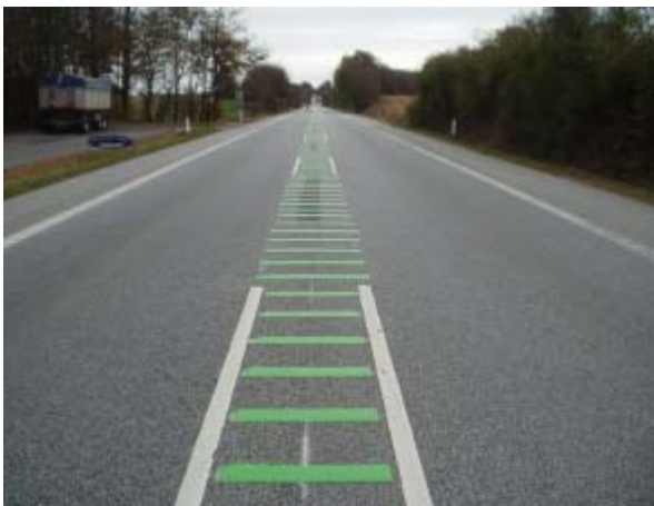
Figure 5.1a: Centre line marking – design A.
