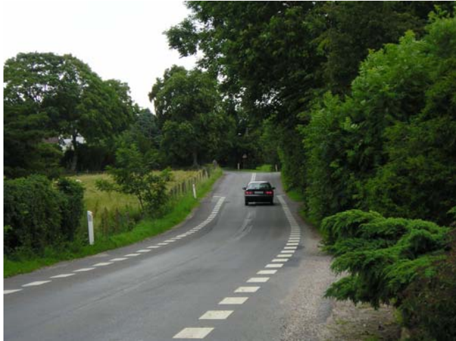
Figure 6.3: Transition from "2-1" rural road to the ordinary two-lane rural road with centre line ahead
