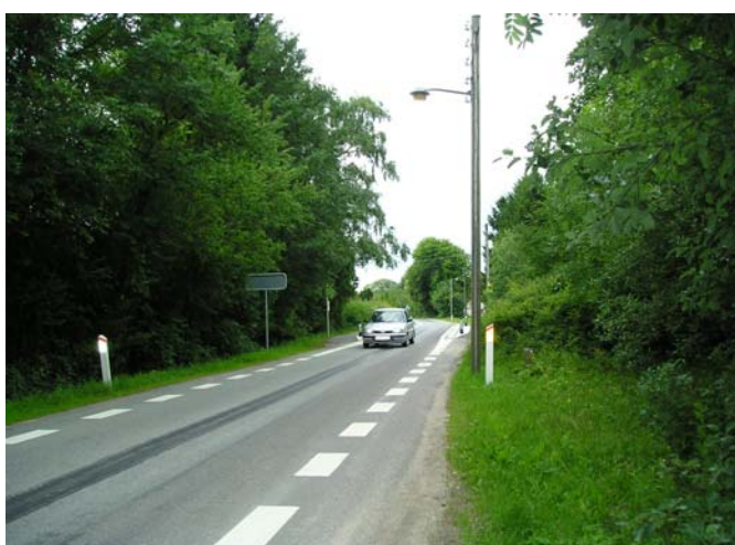
Figure 6.1: "2-1"- cross profile with one central driving lane
