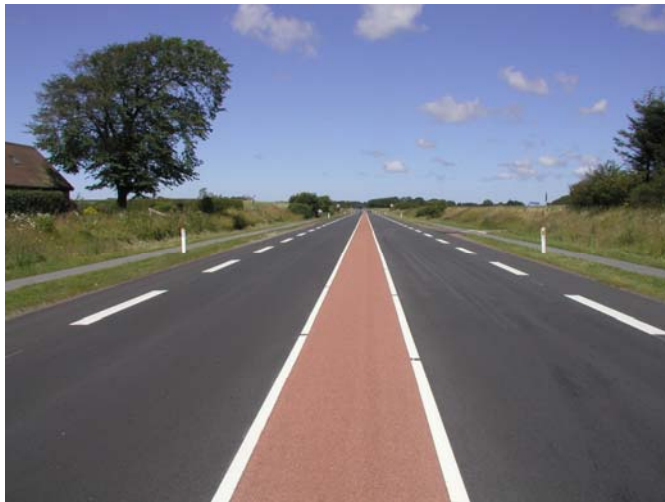
Figure 8.1: Red colored central area flanked by reflectors.
