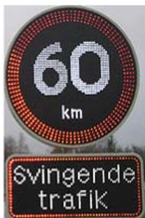
Figure 7.3: VMS sign showing temporary speed limit and warning for crossing traffic ahead.
